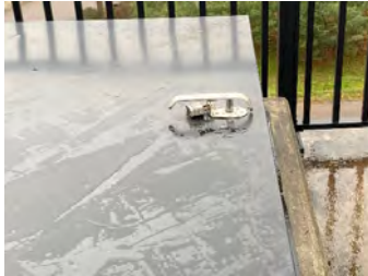
Photo of locked hatch after completion of services
