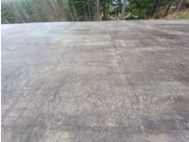
Overall Photo of North Roof Quadrant
