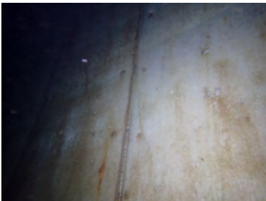
Overall Photo of Interior South Wall Quadrant
