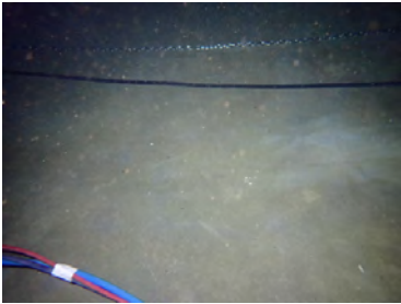
After Sediment Removal
