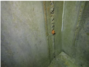
East Wall Aesthetics Photos
