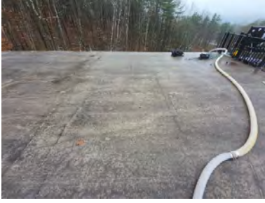
Overall Photo of South Quadrant
