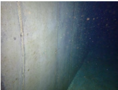
Overall Photos of Interior East Wall Quadrant
