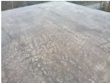
North Roof Quadrant Aesthetic Photos
