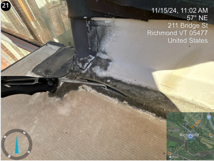
Split in the membrane at a vertical transition.
