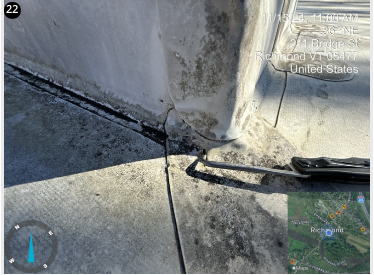
Puncture in curb corner.
