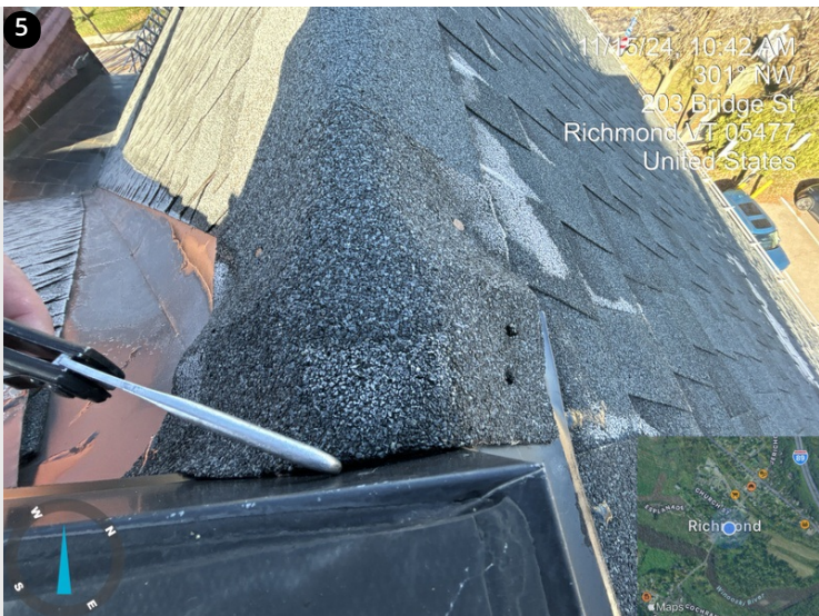
Open area along ridge cap junction.
