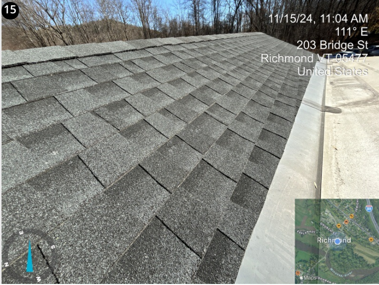
Shingle transition overview.
