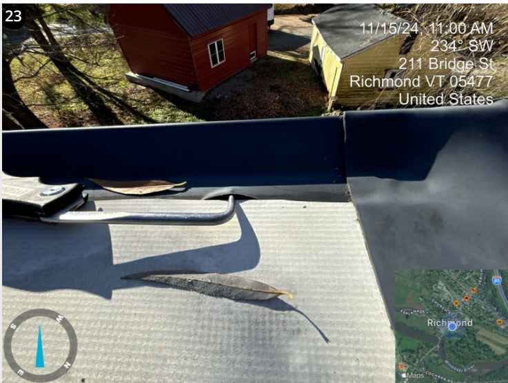
Temporary flashing along perimeter is starting to lose adhesion.
