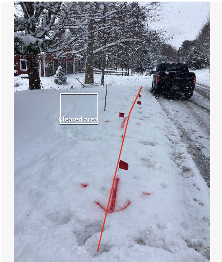
Point #2, Westall rd: Electrical line in close proximity to stake. Recommend moving stake back 3'-5'.
