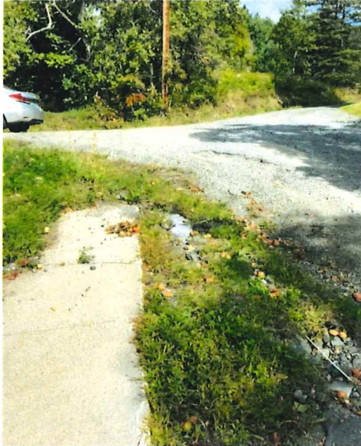
Left: Looking uphill on Folsom Avenue prior to construction. Note failed, undersized culvert to right of sidewalk. Right: Looking downhill on Folsom Avenue during construction. Infiltration basin is north of High Street.
