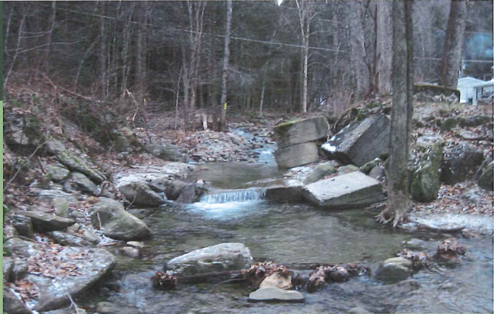
View of old bridge abutments and concrete blocks from downstream (December 6, 2020)
