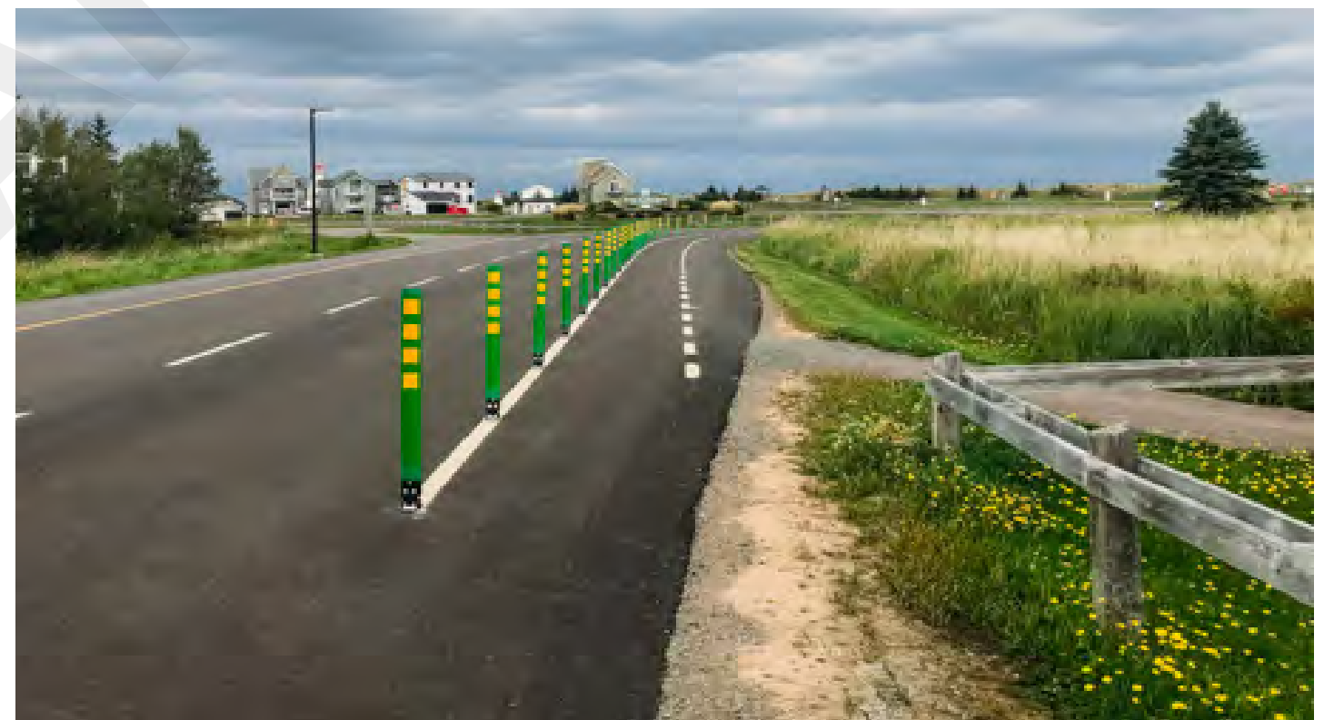
Two-Way Bicycle Lane - Parlee Beach Provincial Park - Shediac, New Brunswick, Canada (delevotech.com)
