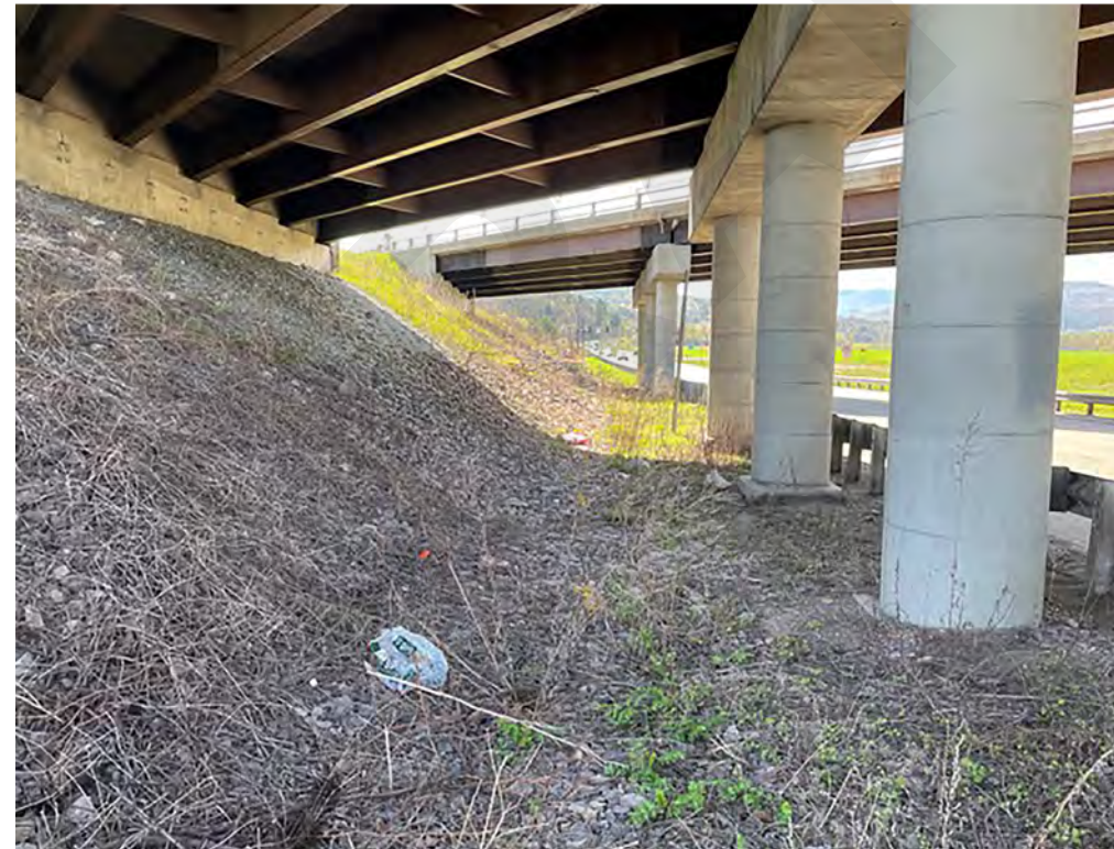
Existing condition under the Interstate at Exit 11 in Richmond.
