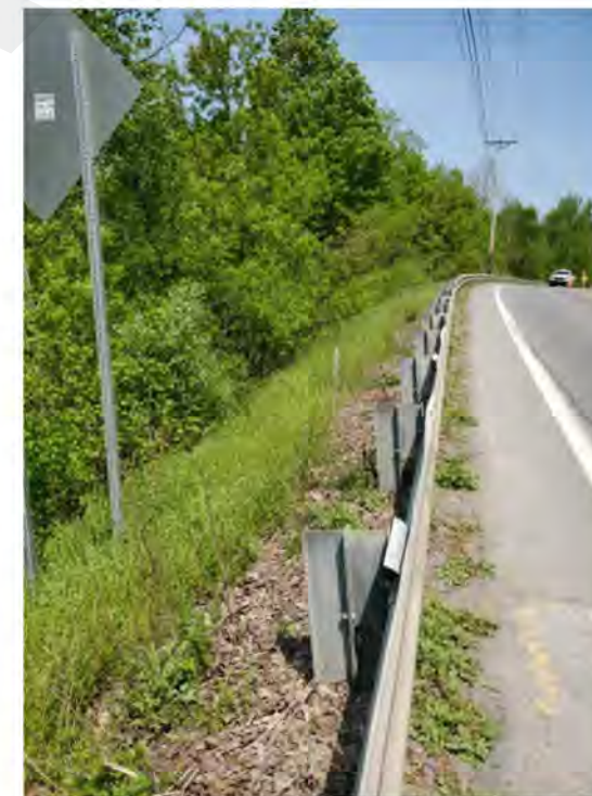
Figure 6: Embankment on US-2 facing west.
