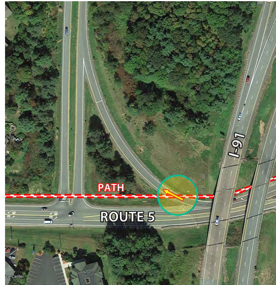
Before: With Slip Ramp at I-91 Exit 11 in Hartford, VT
